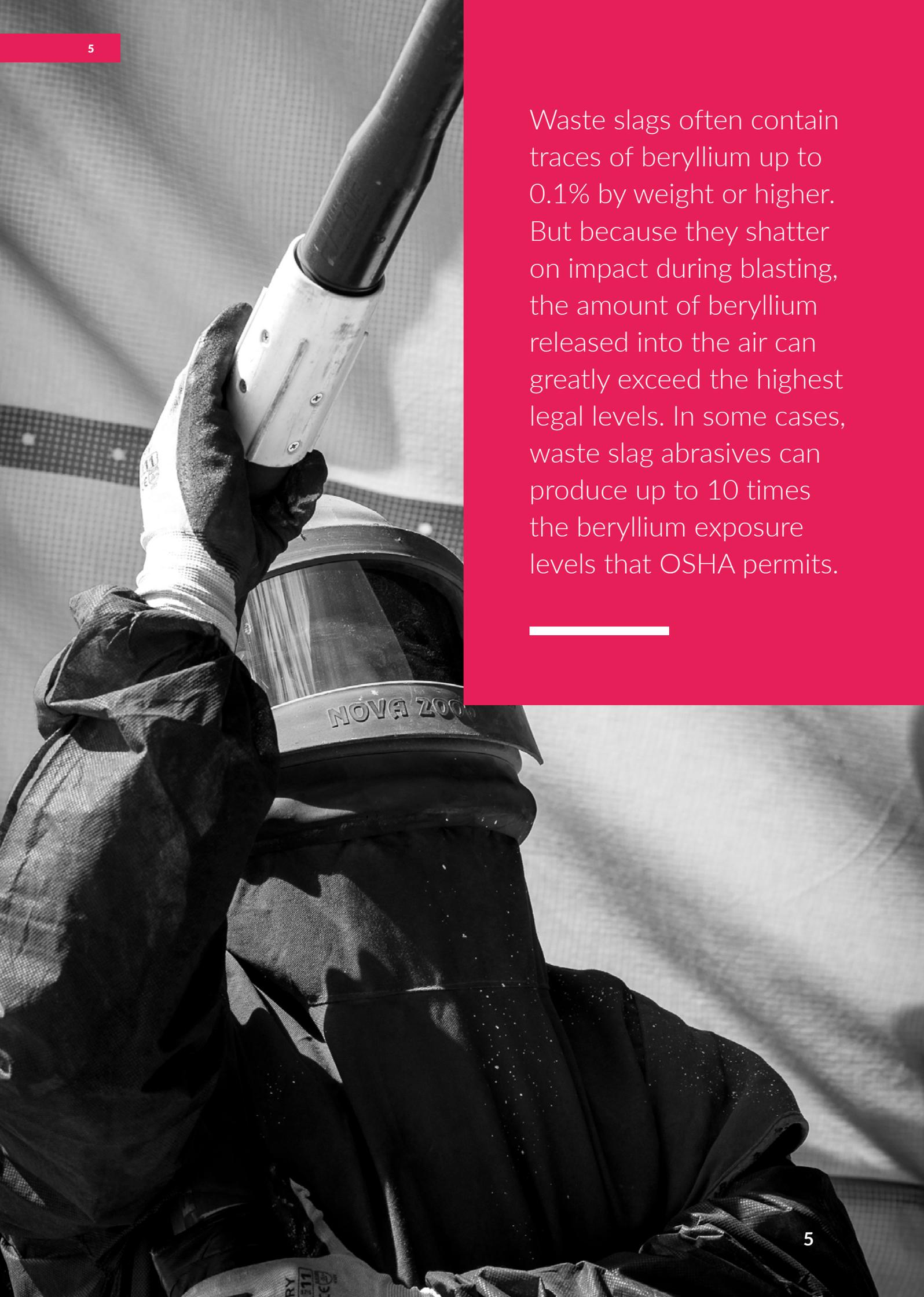
Waste slags often contain traces of beryllium up to 0.1% by weight or higher. But because they shatter on impact during blasting, the amount of beryllium released into the air can greatly exceed the highest legal levels. In some cases, waste slag abrasives can produce up to 10 times the beryllium exposure levels that OSHA permits.
